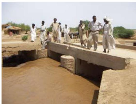
Figure 15 Flow divider at Makala channel, Gash, Sudan.
