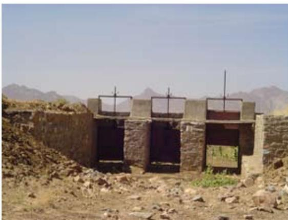
Figure 12 Intakes and sluice gate to improved small system, Alebu (Gash Barka), Eritrea.
