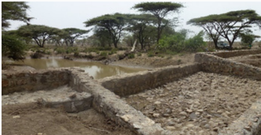
Water Spreading weirs in Afar. Credit: ILRI/Fiona Flintan
