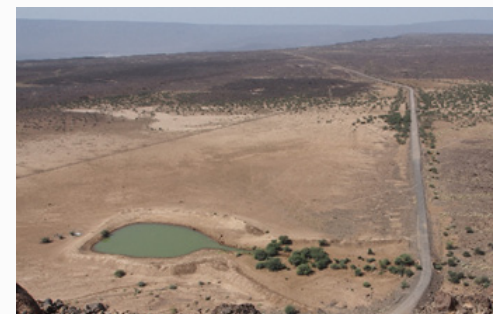
Road water harvesting structure in Afar. Credit: MetaMeta
