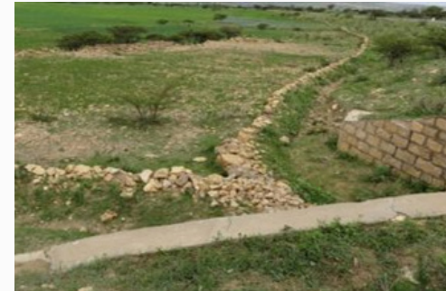
V-shaped diversion structure constructed from soil and stone to spread water from culvert, Ethiopia. Credit: https://roadsforwater.org/
