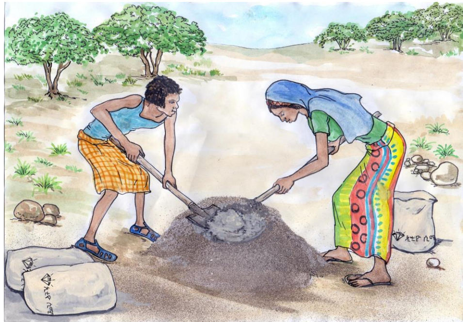
Illustration 23: Sand and cement are mixed.
