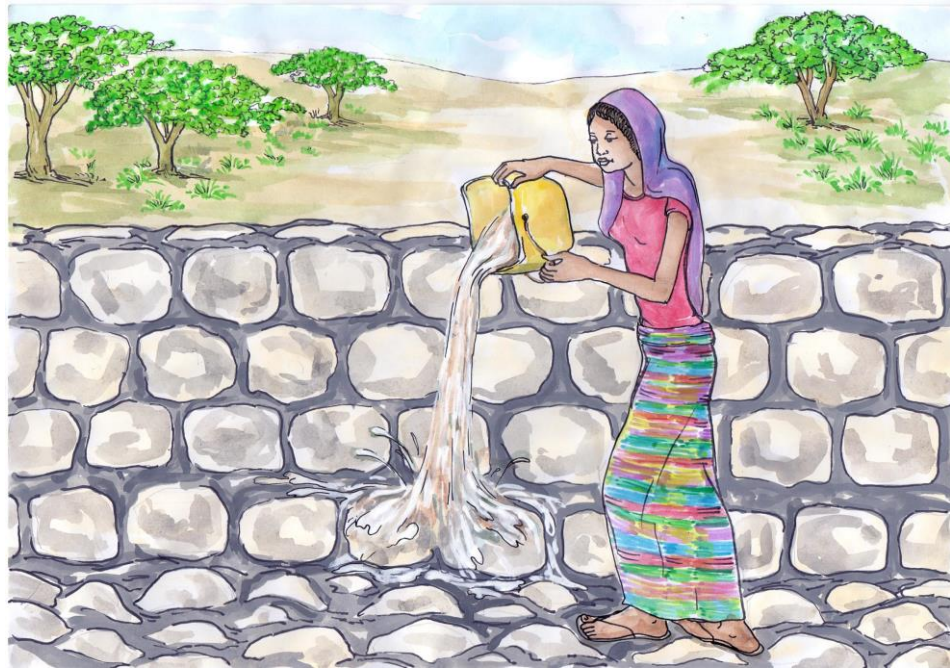
Illustration 28: watering of completed walls is extremely important.
