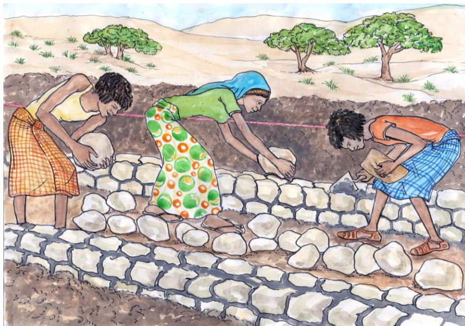
Illustration 25: The counter wall on the left was constructed and the main wall is under way of construction.
