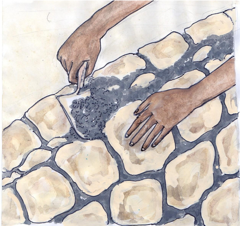
Illustration 31: Lay stones and mortar together at the same time
