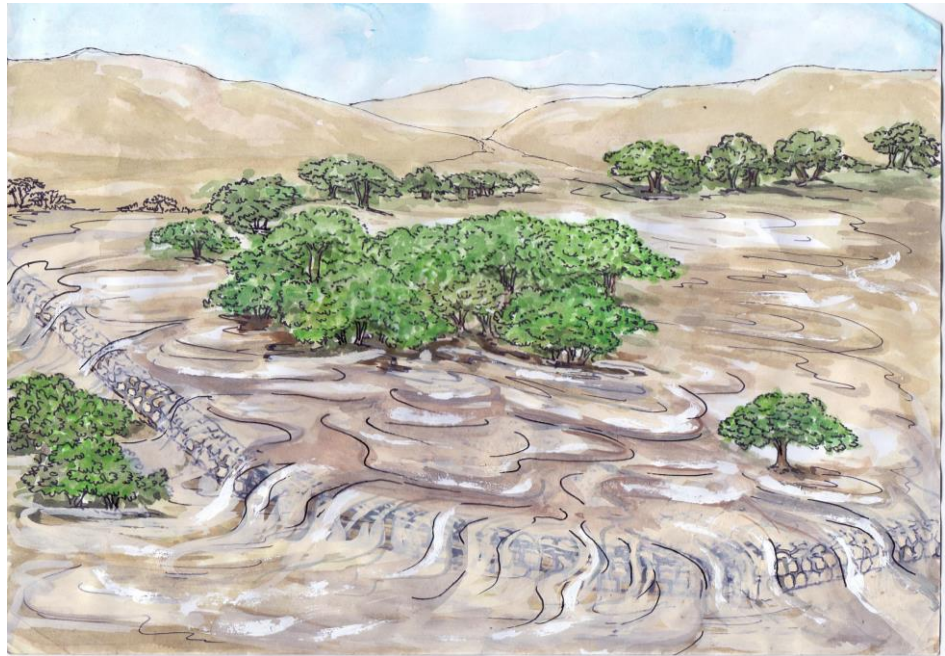
Illustration 8: A Water Spreading Weir is overflown.
