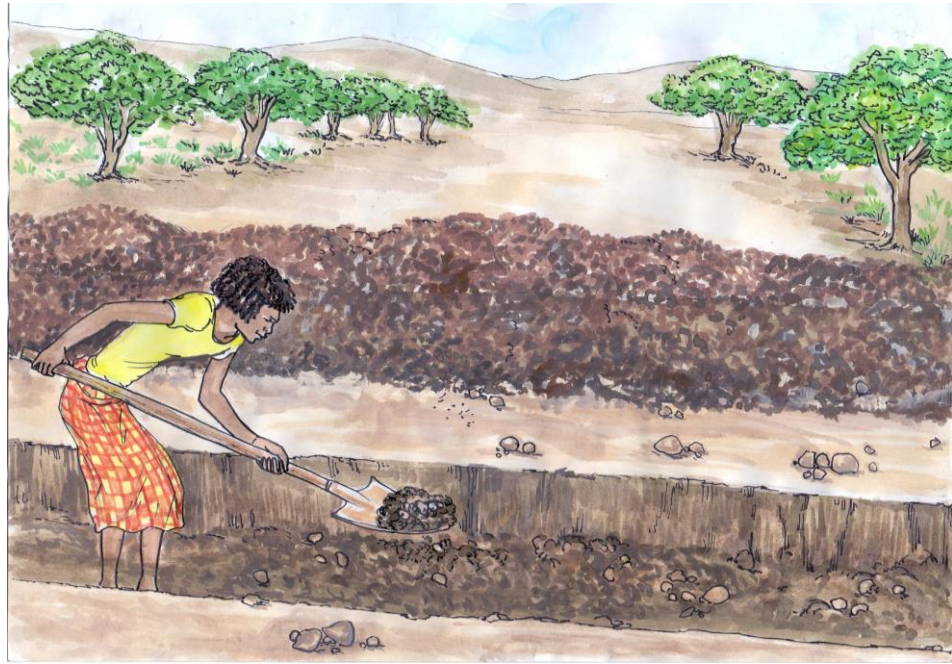
Illustration 22: excavation of the main spillway and basin, with the dry riverbed above.
