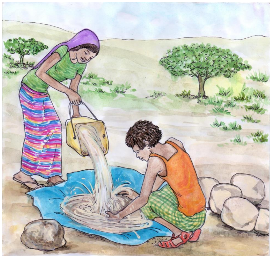
Illustration 29: Remove dirt from stones before constructing with them.
