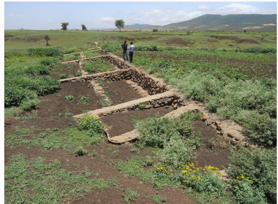
Picture: Water spreading weirs to control erosion and 'plug' the gullies with sediment in Bolidid. Credit: Girma Senbeta
