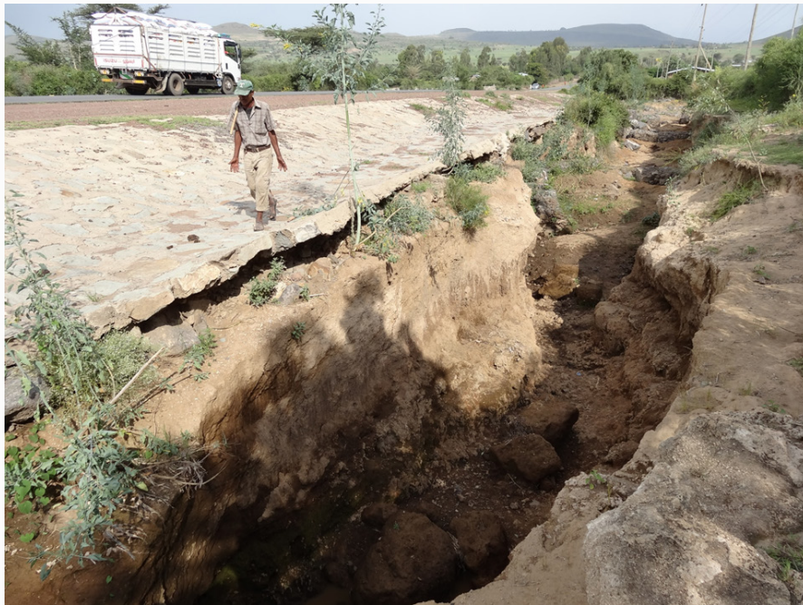
Picture: A gully threatening main traffic road in Boldid area. Credit: Girma S. and Solomon Y.
