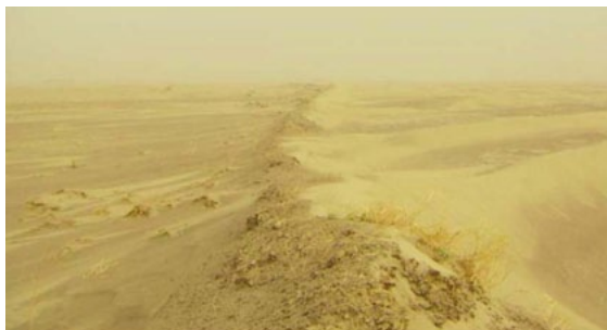
Figure 17: Guide bunds to spread water, sand dunes and depositions impede even spread of floodwater (photo: Ian Macanderson)
