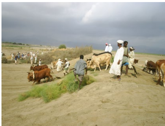
Figure 15: Traditional maintenance of diversion and guide bunds in She'eb scheme (van Steenberg et al. 2011)
