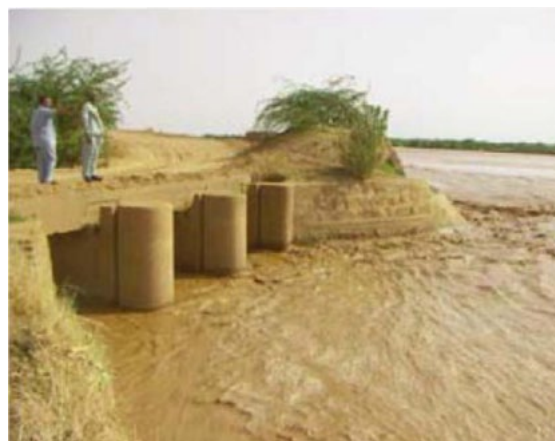
Figure 16: Fota intake, silt-laden floodwater, Gash scheme (van Steenberg et al. 2011)
