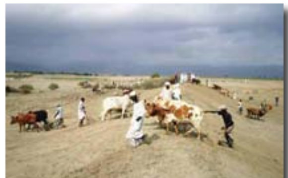
Figure 2.3: Traditional bund intakes in Eritrea
