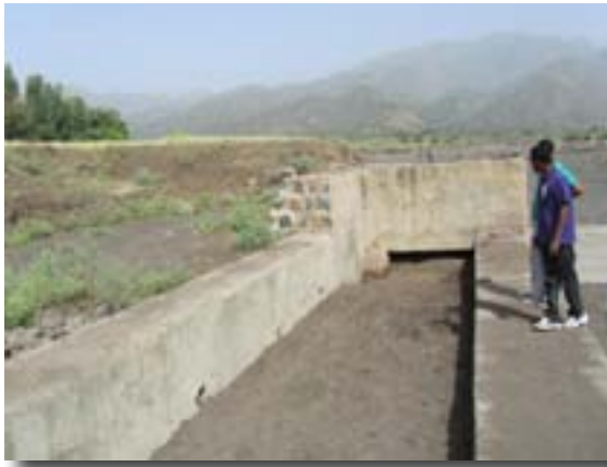
Figure 4.23 Sedimentation problems at the Hara off-take and Fokisa canal systems
