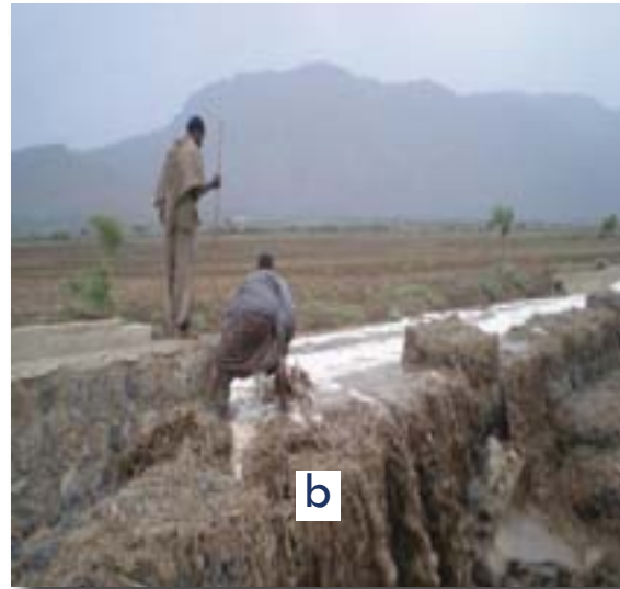
Figure 4.25 A zigzag canal in traditional systems (a) and breach by retreating flood in straight canals (b)
