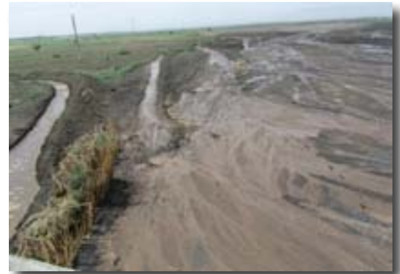
Figure 4.20 The Harosha traditional spate system having many diversion points along the Wadi at an immediate downstream of a bridge
