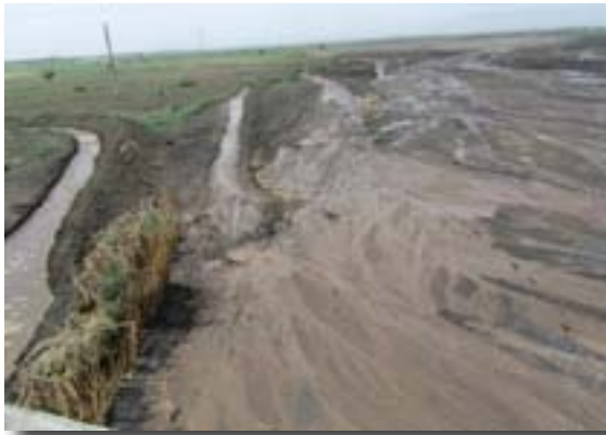
Figure 4.20 The Harosha traditional spate system having many diversion points along the Wadi at an immediate downstream of a bridge
