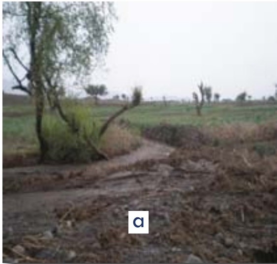
Figure 4.25 A zigzag canal in traditional systems (a) and breach by retreating flood in straight canals (b)
