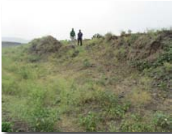
Figure 4.21 Traditional diversion canal at downstream of Dayu spate scheme left over because of Wadi bed level lowering
