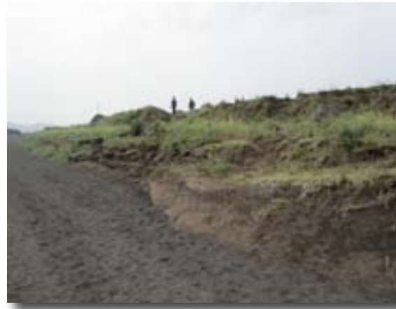
Figure 4.21 Traditional diversion canal at downstream of Dayu spate scheme left over because of Wadi bed level lowering
