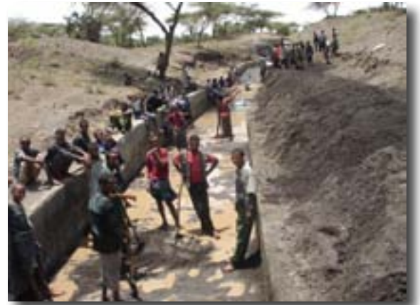
Figure 4.23 Sedimentation problems at the Hara off-take and Fokisa canal systems
