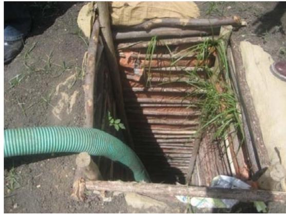
Figure 8-9: Hand dug well constructed around Koka dam
