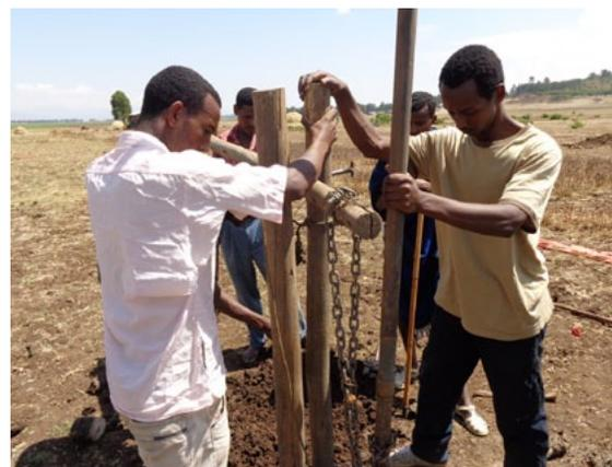
Figures 15-16: Installing sludge drill in Fogera plain
