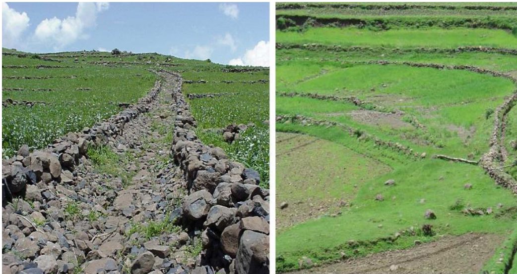
Photo 5: Waterways for disposing discharge coming from cutoff drains and graded terraces (Photo , 2004)
