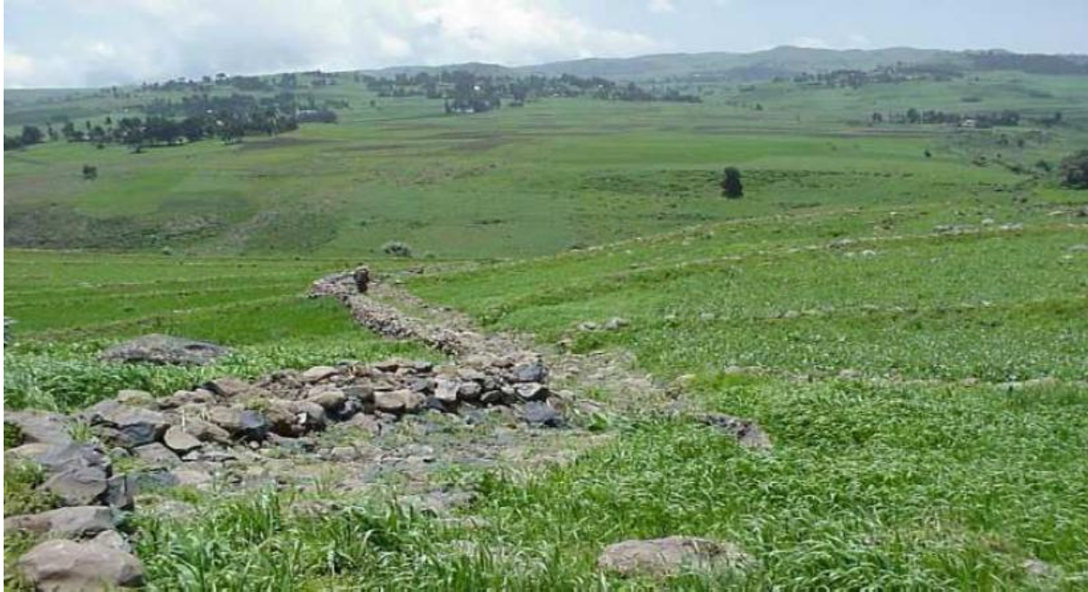
Photo 6: A waterway constructed to convey runoff from terraces and cut-off drains
