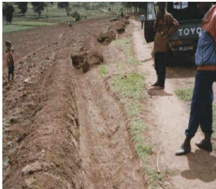
Photo 1: Cut-off drain leading to a waterway
