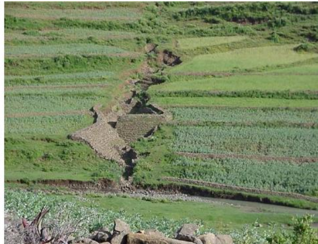
Photo 8: A natural waterway stabilized by stone riprap and farm check dams
