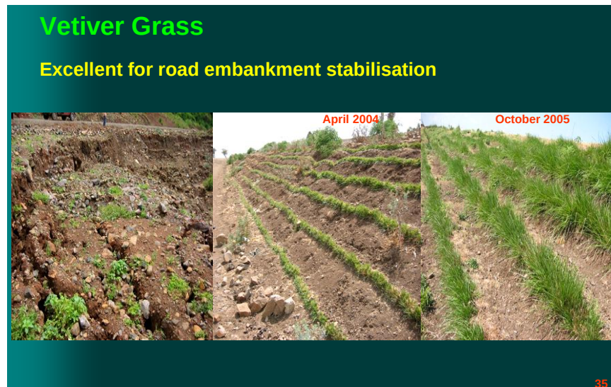
Figure 19: Vetiver grass for road embankment stabilization
