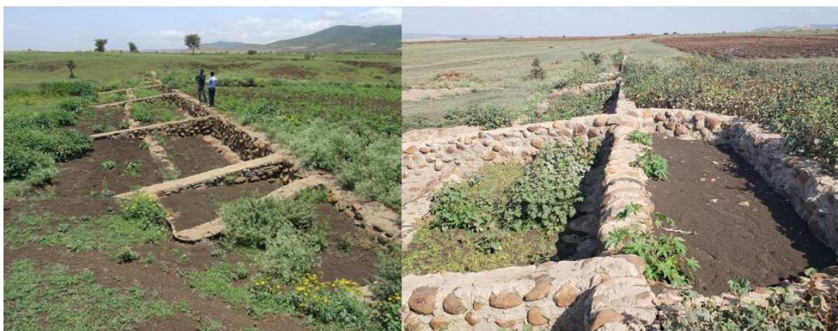
Figure 9 Water spreading weirs in Bolidid and Karamara (Pictures by Girma Genbeta)
