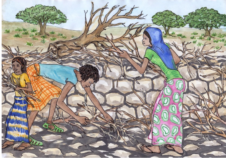
Figure 26: Covering the constructed WSW to ensure good curing
