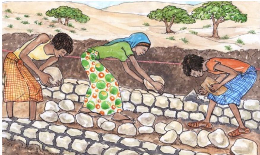
Figure 18: Constructing the main wall
