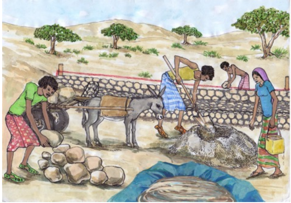
Figure 13: Construction site for a Water Spreading Weir
