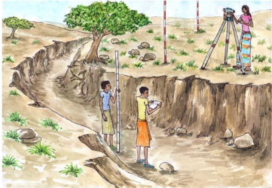
Figure 7: Setting out the WSW
